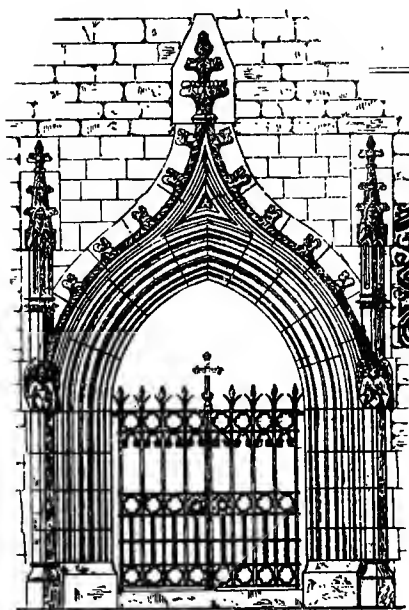
SOUTH ARCHWAY TOWER, ST. JOHN'S CHURCH, CARDIFF.
